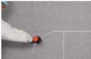
Removing groove lines.
