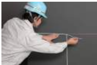
Fixing joint material.
