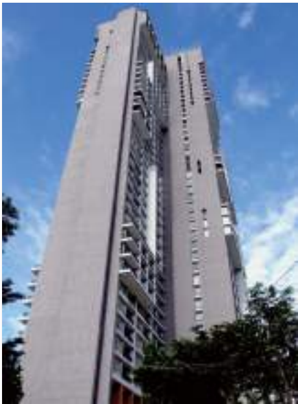
Issara Lard Plao Condominium (Thailand)
